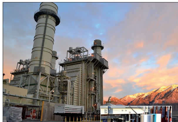
The Combined-Cycle Generation Power Plant in Western USA
