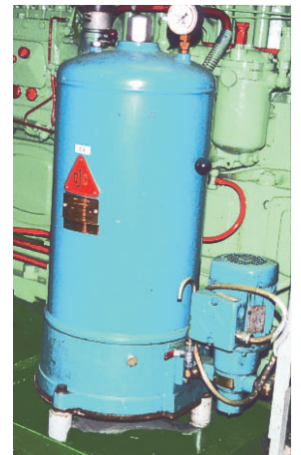
HDU2 27/54 P for lube oil treatment.
