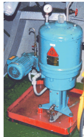
PTU2 27/27 P. for gas oil separation.
